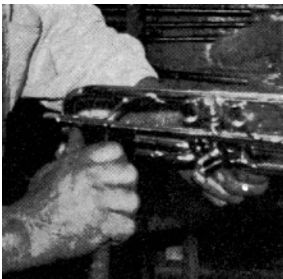
In finishing a solder job, the hook scraper is used to reach those parts not easily accessible.
