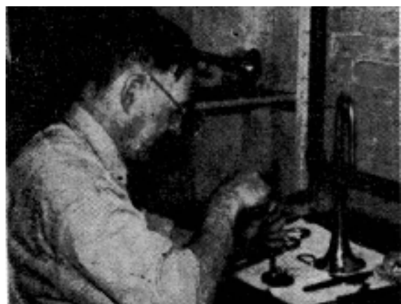
Sinking curved patch in lead block.
