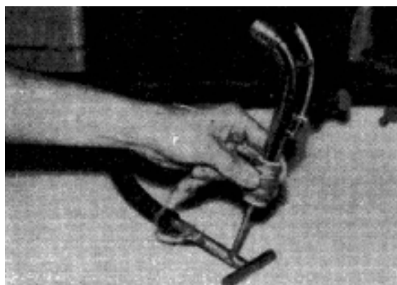
Applying flame inside neck to melt shellac to cause cork to adhere.
